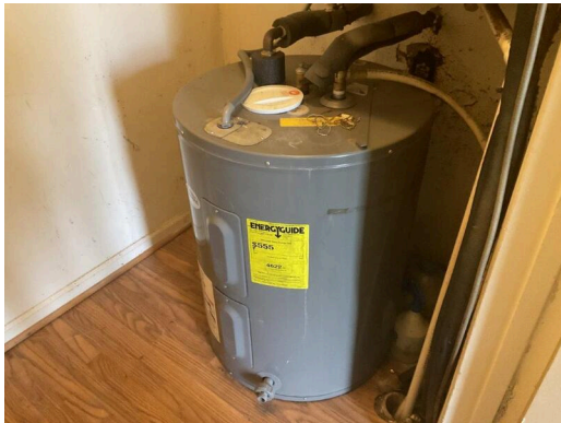
PHOTO #27 ELECTRIC WATER HEATER
