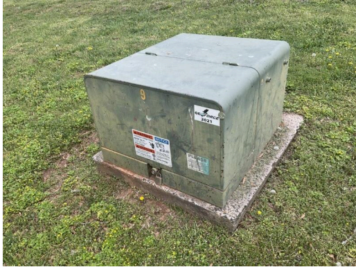
PHOTO #25 PAD-MOUNTED TRANSFORMER
